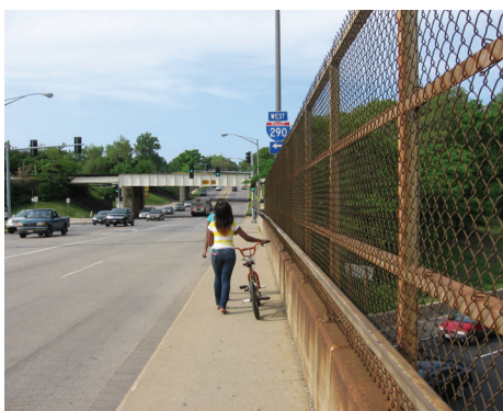
A cyclist walks her bike over the Des Plaines Avenue Bridge.
