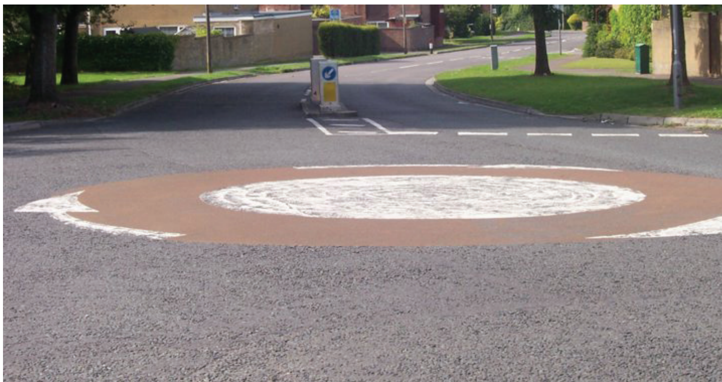
A mini-roundabout can further help to calm traffic at confusing 5-way intersections.
