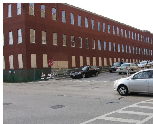
Circle Avenue Bridge from Harrison Street
